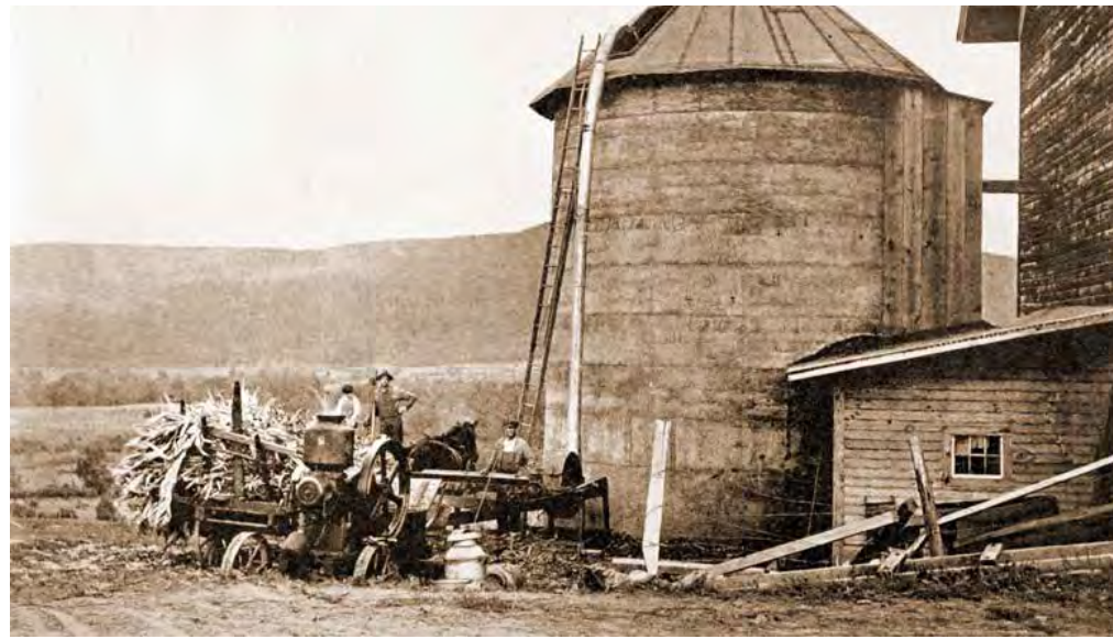
Cutting ensilage and filling the silo
