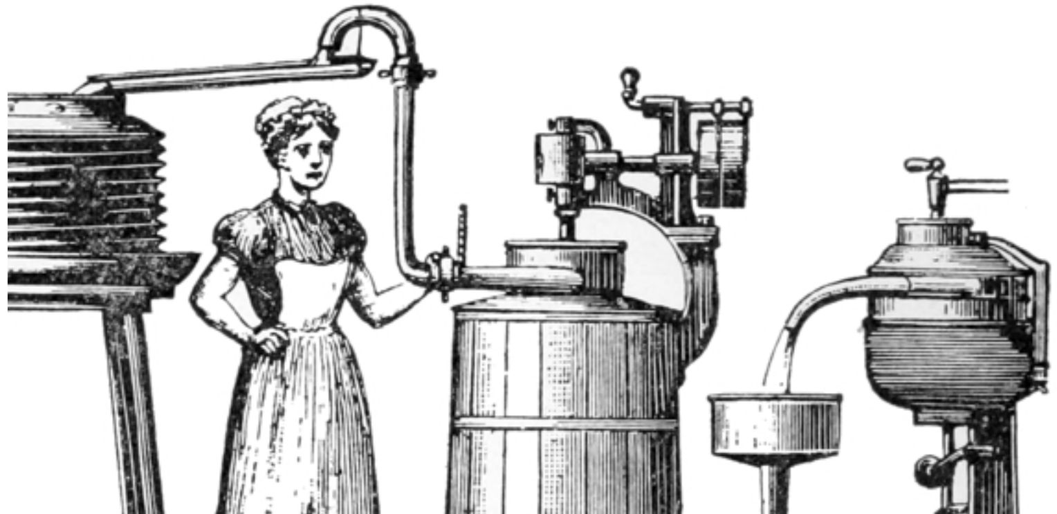
Installation in a Danish creamery. From the separator at the right the cream runs through the continuous pasteurizer which forces it up over the cooler whence it runs into the cream-vat at the left. (From Boggild—Maelkeribruget i Danmark)
